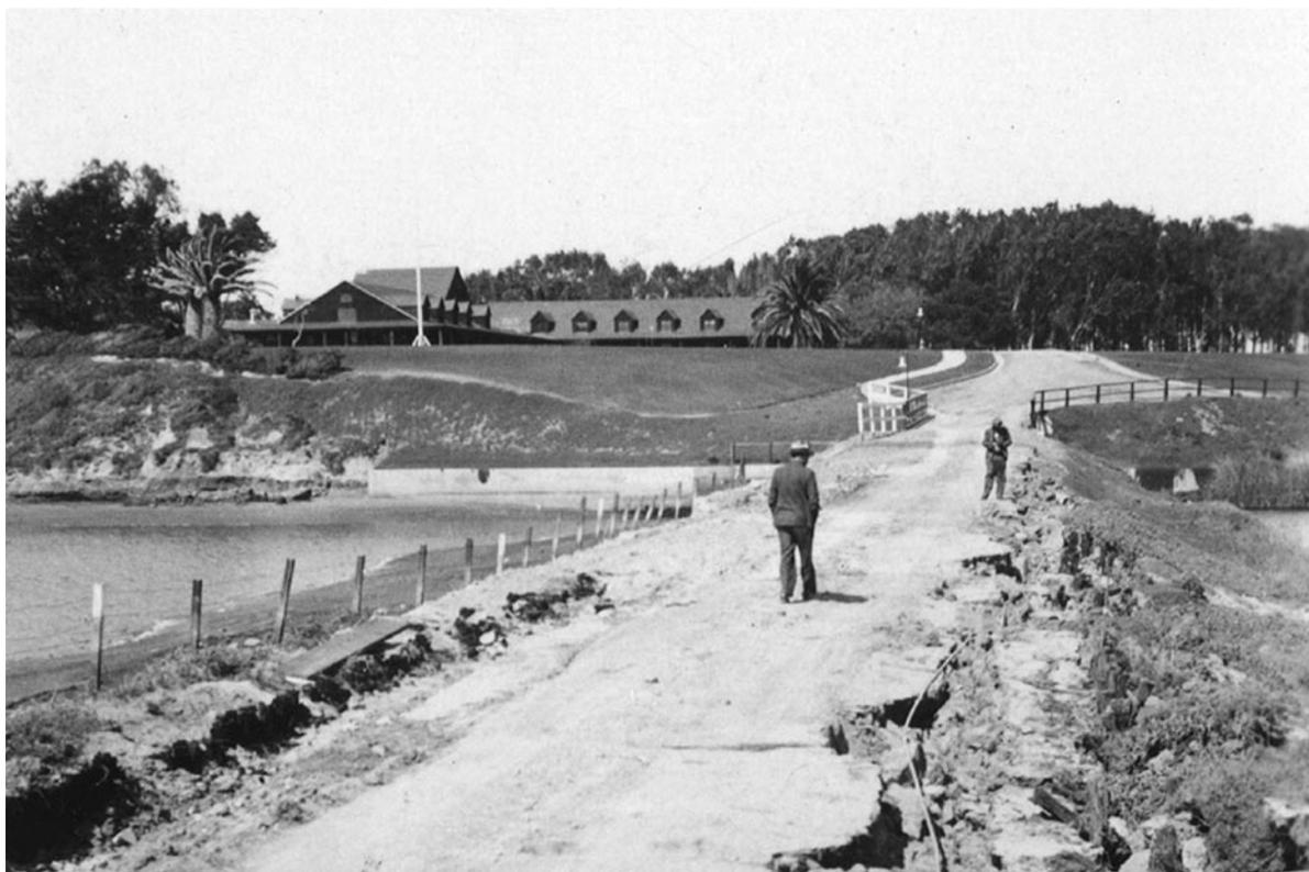
Figure 9. Bolsa Chica Gun Club (BCGC). Photograph taken by W. W. Bradley shortly after the Long Beach earthquake of March 10, 1933. Note damage along both sides of the dam. The dam was constructed for the BCGC by Tom Talbert to prevent tidal flow from entering into the wetlands east of the dam. This barrier enabled the BCGC “to construct duck ponds about the property and enjoy calm hunting waters” (Carlberg 2009:71). Courtesy U.S. Geological Survey Photographic Library.
